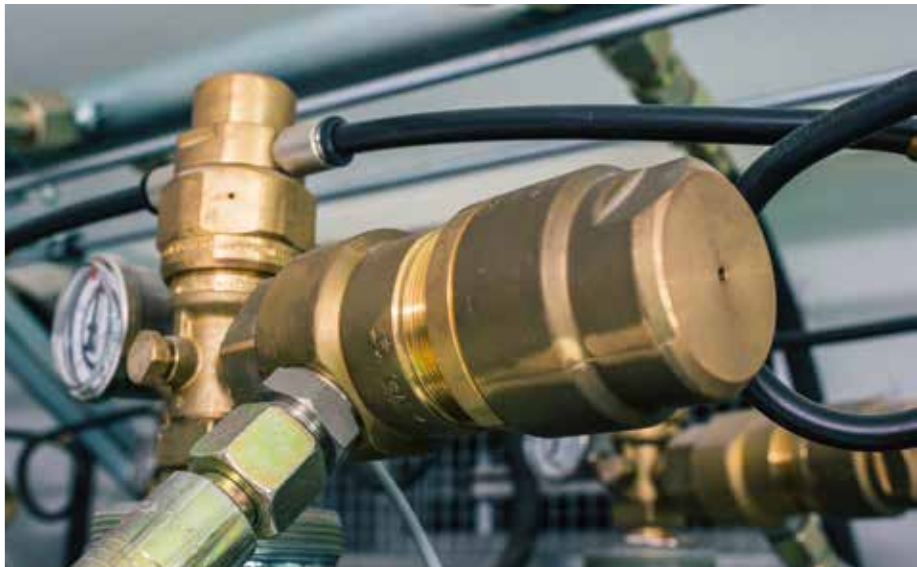
Flow regulator for soft flooding
